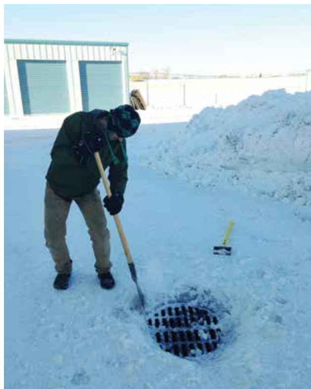
Iced up storm drains must be dealt with. Having the right tools on hand is important. (Photo courtesy of Randy Schubert)
