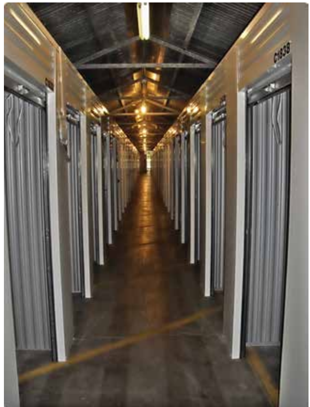
Janus International form-fitted sheet metal to each wall to convert the caves into modern self storage units.
