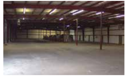
Above: A warehouse formerly used by a moving company in Matthews, North Carolina.
