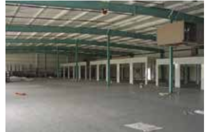
Below: Showing the conversion into a self storage facility by BETCO.
