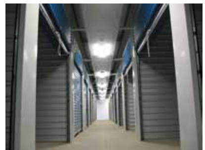
Above: Miller Building did this conversion at what is now Glenolden Storage Center in Glenolden, Pennsylvania.
