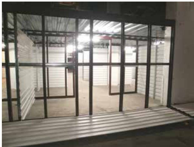
Work being done by Paramount Metal Systems creating a Storage Plus in Brooklyn, New York.
